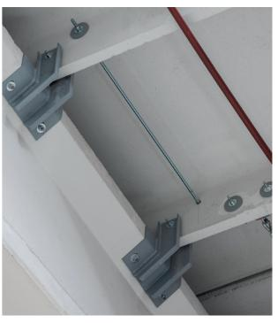
Examples of roof-beam constraint systems
