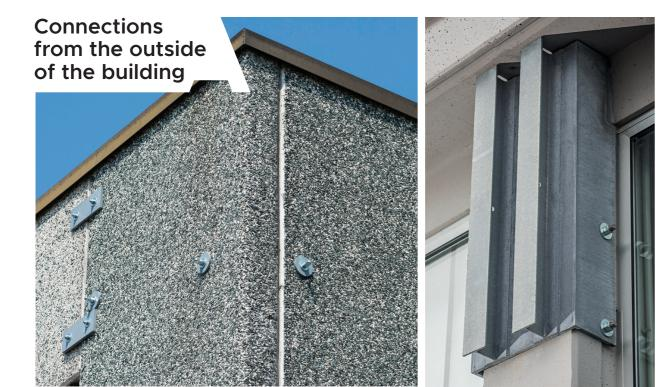
Examples of externally installed constraint systems
