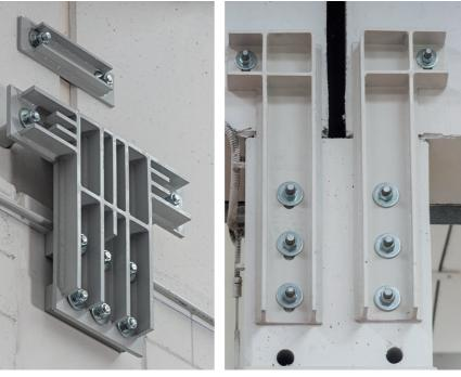
Examples of beam-pillar constraint systems
