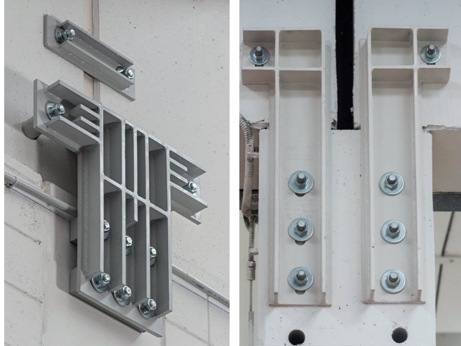
Examples of beam-pillar constraint systems
