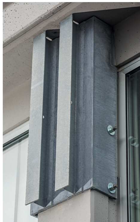
Examples of externally installed constraint systems
