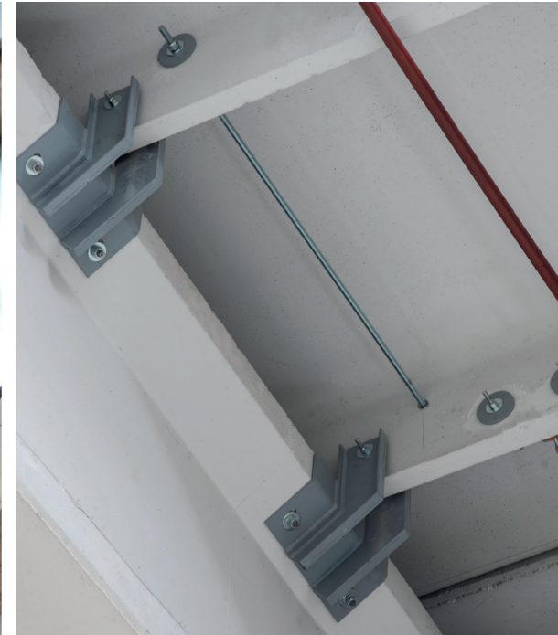
Examples of roof-beam constraint systems
