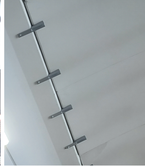
Examples of secondary elements constraint systems
