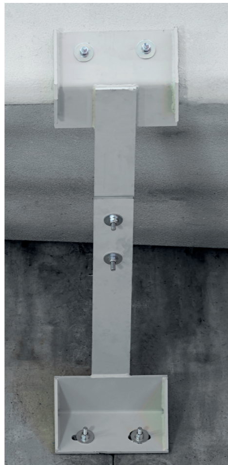
Examples of panel restraint systems
